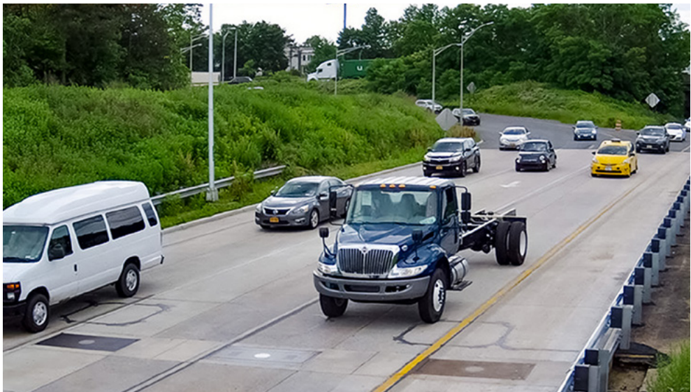
Figure 6: WIM system in advance of the Goethals Bridge in New York, U.S.A.
