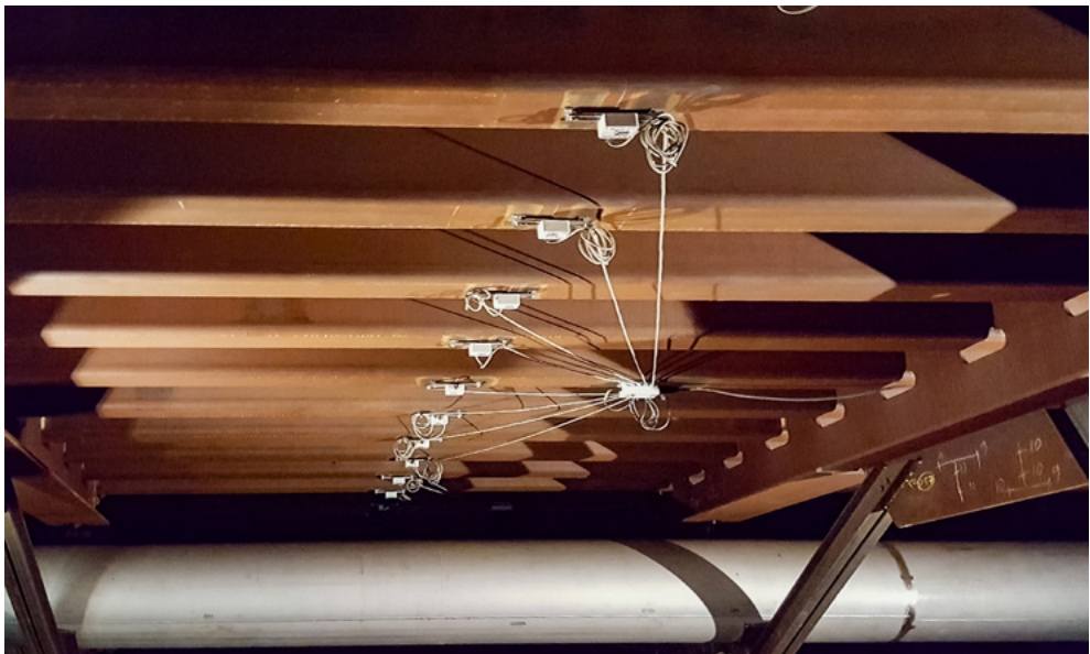
Figure 9: B-WIM sensor installed on one of the spans of the Millau viaduct
