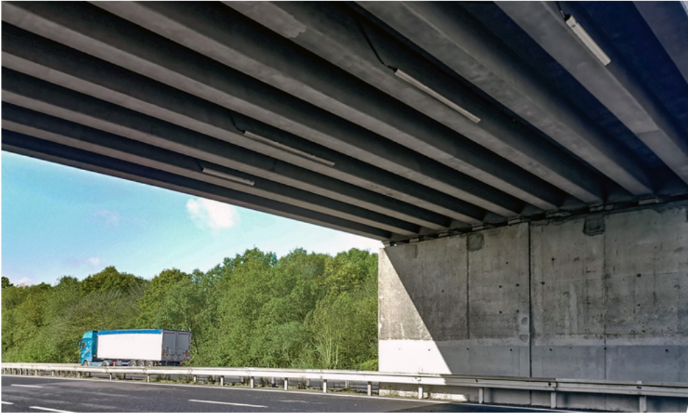
Figure 10: B-WIM sensors on A10 bridge (France)
