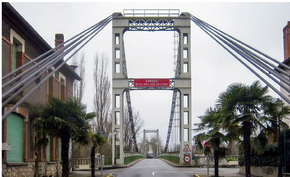
Figure 5: Bridge posted with 19 t limit and not more than one truck. It collapsed when crossed by a 51 t truck.
