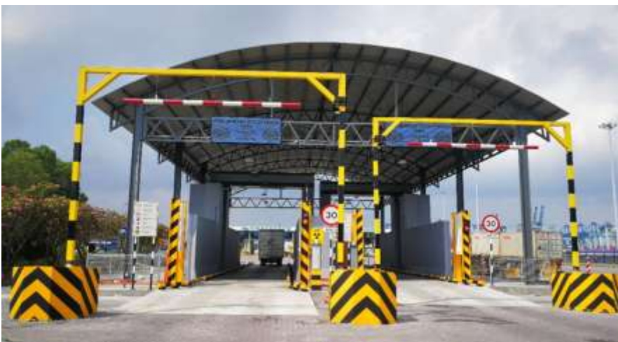
WIM system at the Tanjung Kupang Checkpoint, Malaysia
