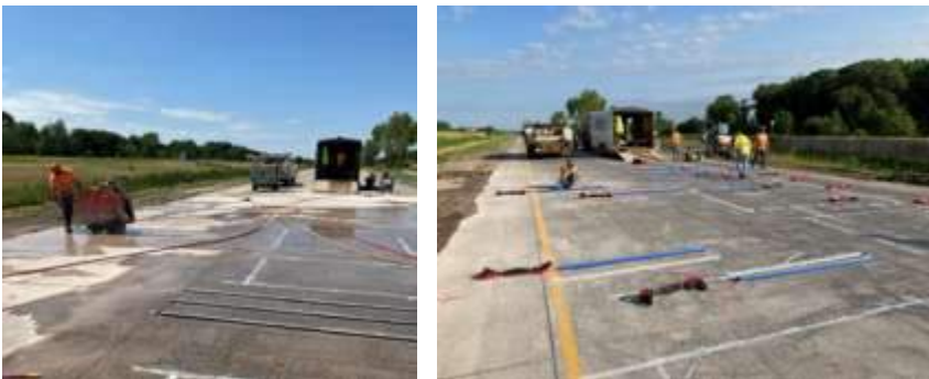
VectorSense and Quartz Sensor Installation
