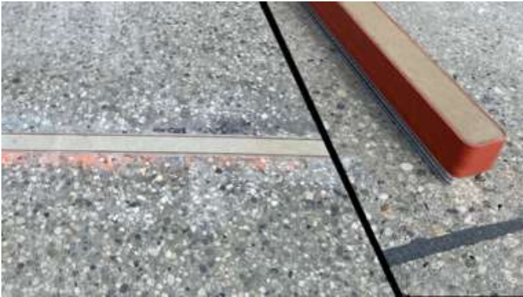
Detail of the installed Strain Gauge Strip Sensors
