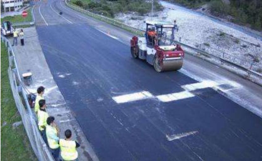
**Resurfacing without removing the BISON bending plates.**
