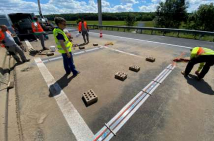
Installing the Lineas sensors on the A6 motorway in Luxembourg
