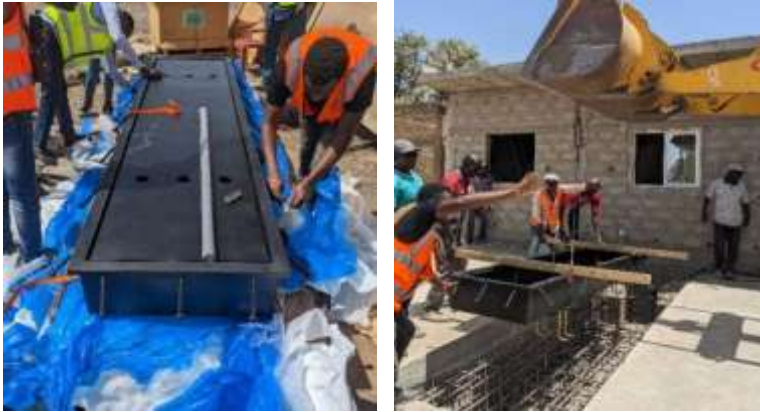
Unpacking the WIM Scale and Installing it at the Facility Entrance
