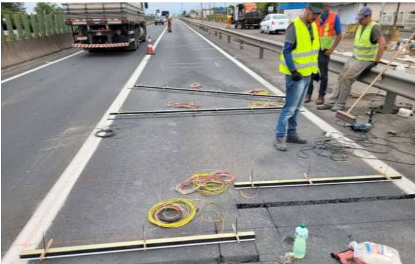
Installation of the CAMEA HS-WIM on the BR-101 highway.
