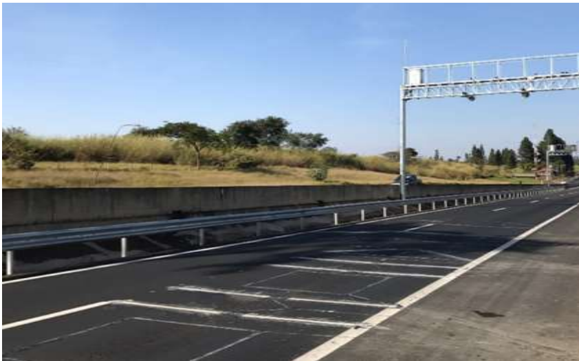
HS-WIM system type-approved for direct enforcement in Brazil
