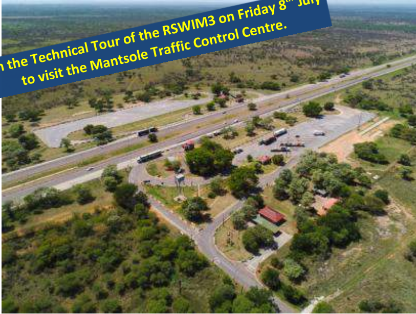
Aerial View of the Mantsole Traffic Control Centre
