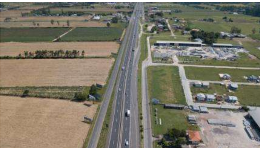
WIM Test site at Araranguá, highway 101, Santa Catarina, Brazil.
