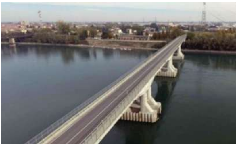
One of the many bridges in Italy monitored by a iWiM BISON system
