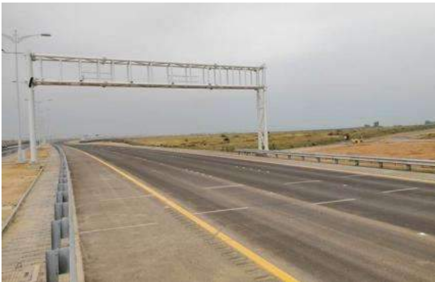
Intercomp's new Microstrip™ sensor installed in a US highway.
