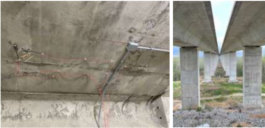
NOR Bridge WIM system installed in Virginia, USA.
