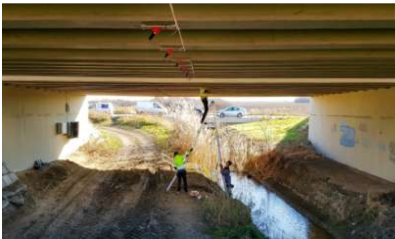
Installation of a Cestel Bridge WIM system in Serbia.
