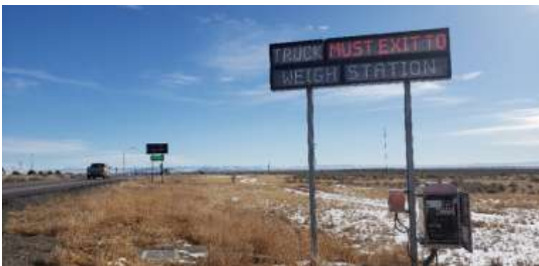
iSINC® WIM Electronics and CMS at the eastbound WIM location
