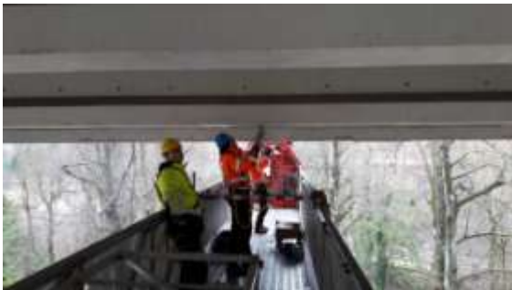
Installation of the SiWIM sensors under the bridge.
