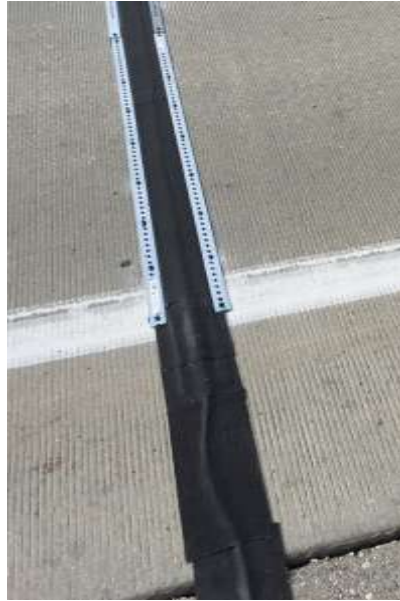
Portable WIM sensor installation
