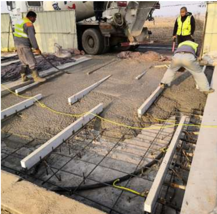
VanJee staff installing digital bar sensors in China.
