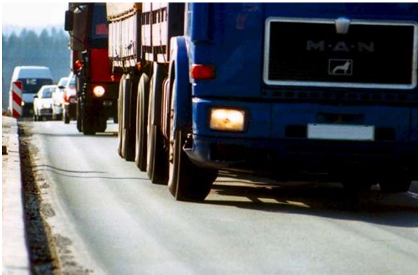
Figure 5: Severe rutting in road pavement
