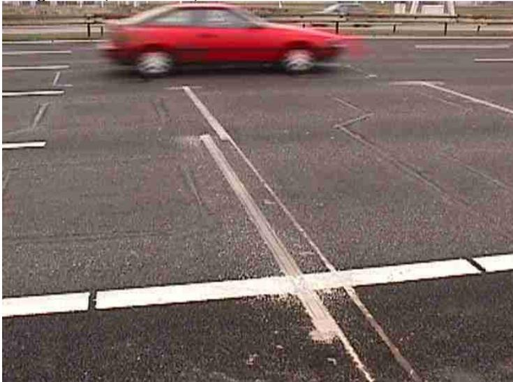
**Figure 2.2, Example of strip sensor**
