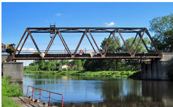
Fig. 1 - Nieporeț Railway Bridge
